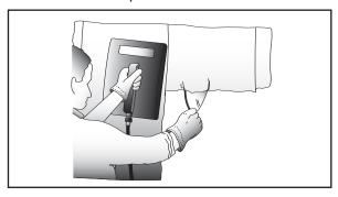
immediately next to where you have just been working and use a wallpaper scraper to remove the section that has just been steamed. By working in this way you should be able to remove paper continually. You may have to leave the plate against the wall for longer periods with some papers or re-steam if not completely removed.
